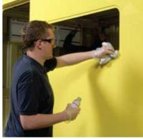
Above: Apply BETAWIPE with a continuous movement to clean and activate surfaces as part of a complete adhesive system.
