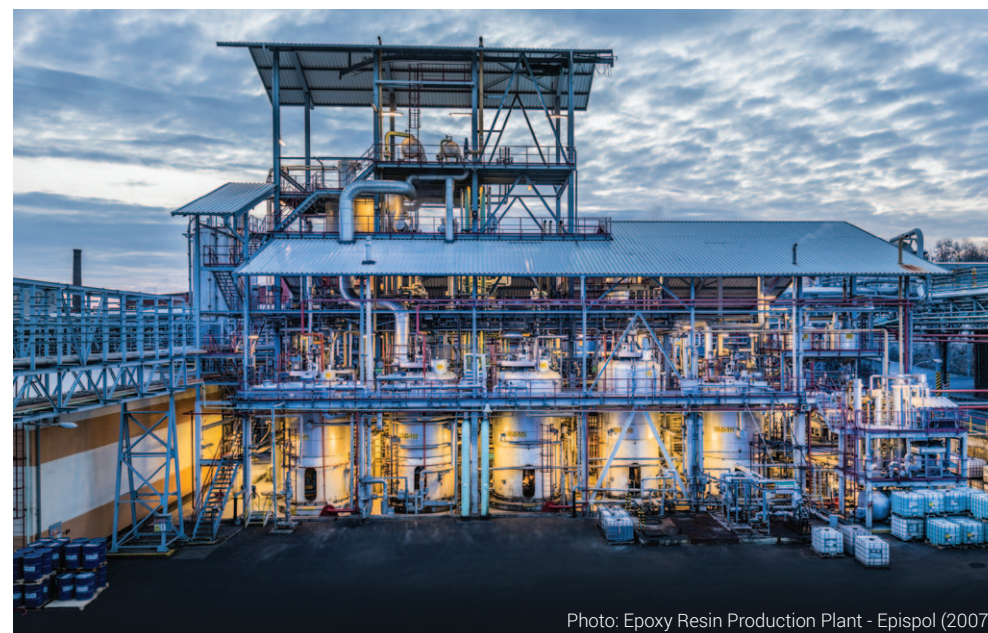
Photo: Epoxy Resin Production Plant - Epispol (2007)
